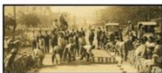
Street construction in Strawn using Thurber bricks. Courtesy W.K. Gordon Center Special Collections
