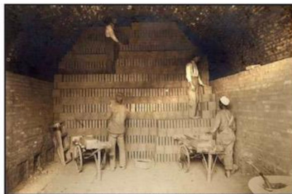
Workers stacking bricks in a kiln where they are to be dried and fired. Courtesy W.K. Gordon Staff
